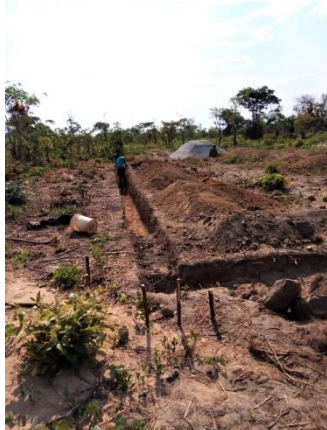
Footer for the new school building
