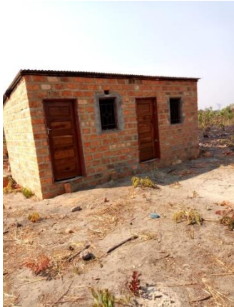
Building for storage and night watchman
