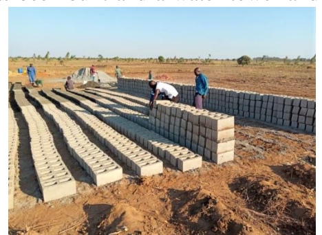
Making your own concrete blocks is a lot of work
