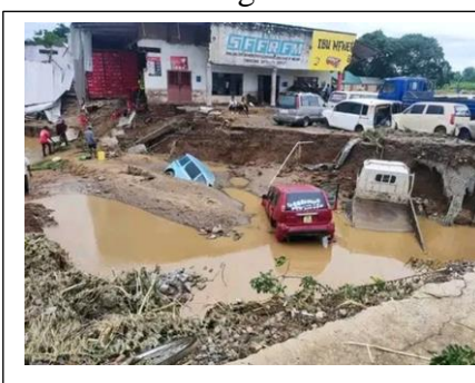
Flood damage Malawi
